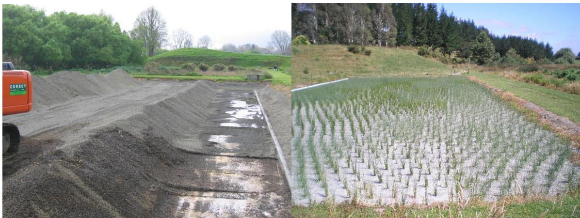
Fig. 2. Vegetated submerged bed wetland.
