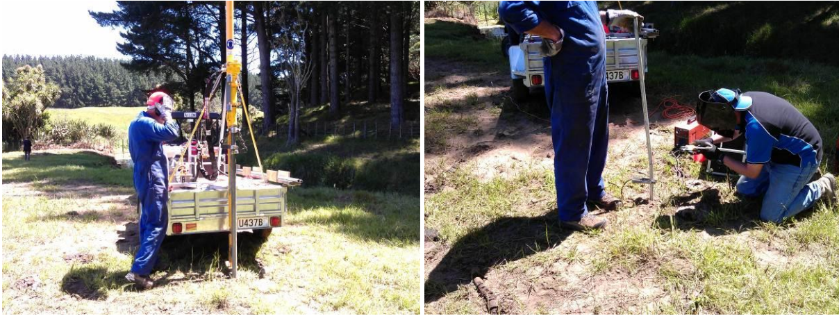
Figure 1 and 2: Standpipe installation.
