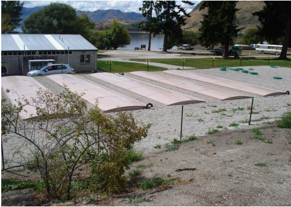
Figure 1: Photo showing Completed System
