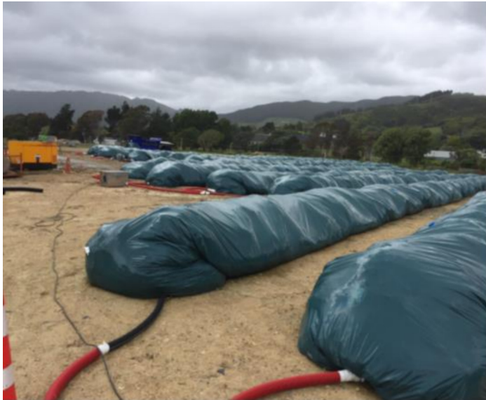
Fig. 2. Geobag trial at Paraparaumu Wastewater treatment plant on the Kapiti Coast
