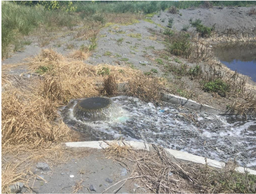
Figure 11: Infiltration Basin Inlet
