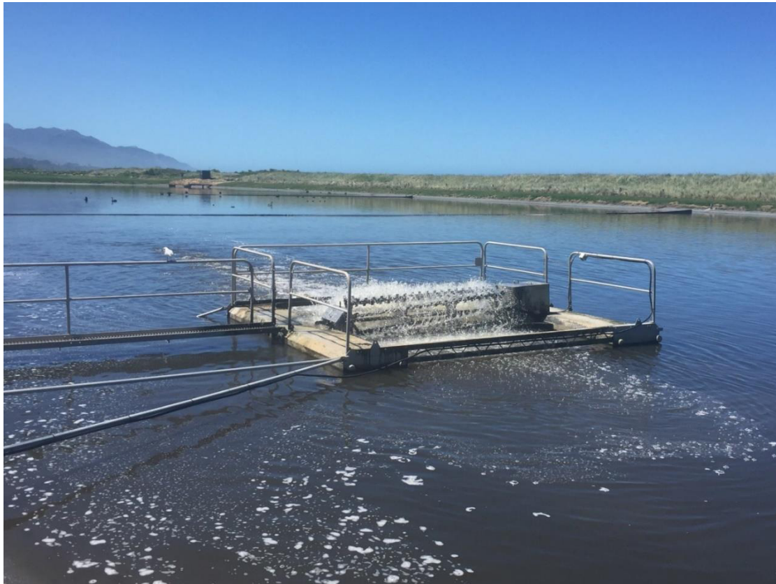
Figure 9: Oxidation Pond Caged Rotor – no Algae
