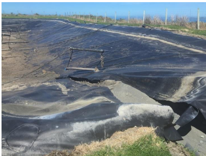
Figure 1: Damaged Aerated Lagoon
