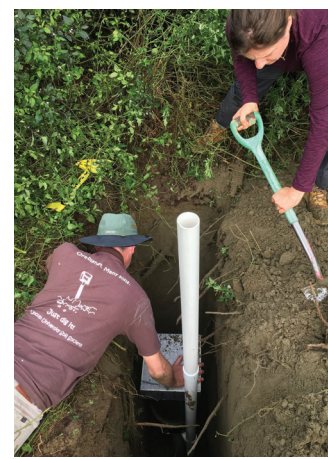
Alexandra Meister and Brett Robinson installing a Water Flux Meter in the Pot experimental site
