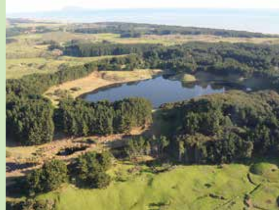
Aerial view of 'The Pot' wastewater pond at Levin (photo credit Sian Cass)
